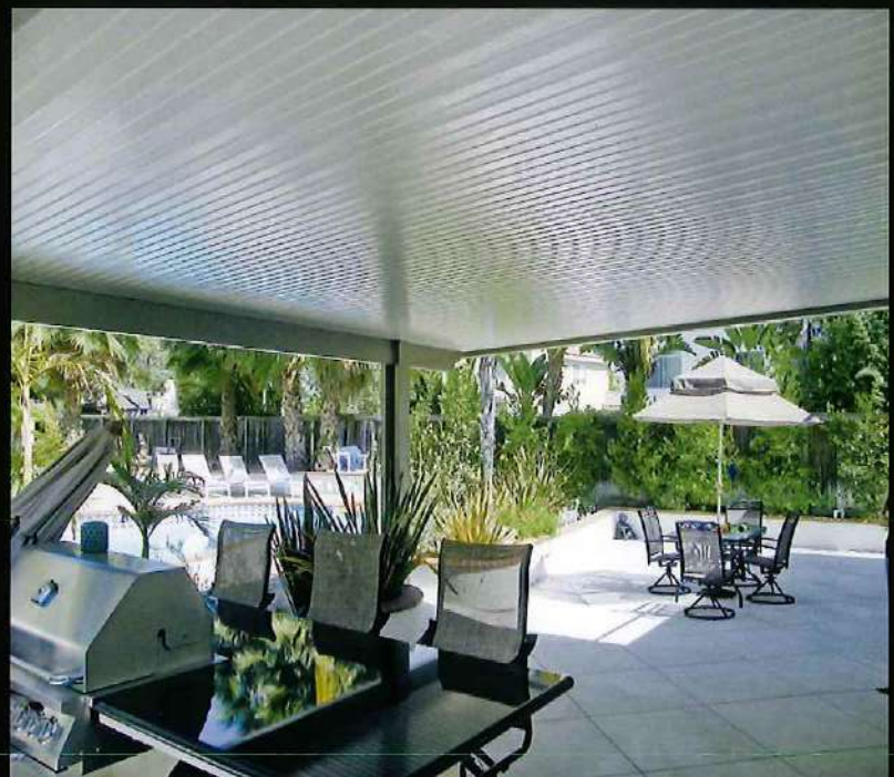
Alumawood flat pan, 2x6 wrap, no tails, 3x8 beam single, and standard post wraps.
