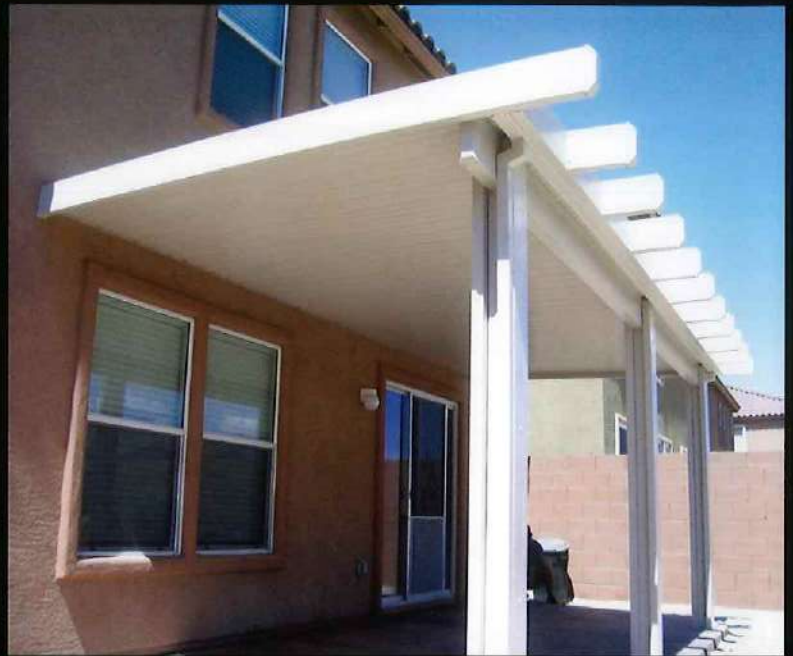
Alumawood flat pan, 2x6 wrap, tails, 3x8 beam, and standard post.
