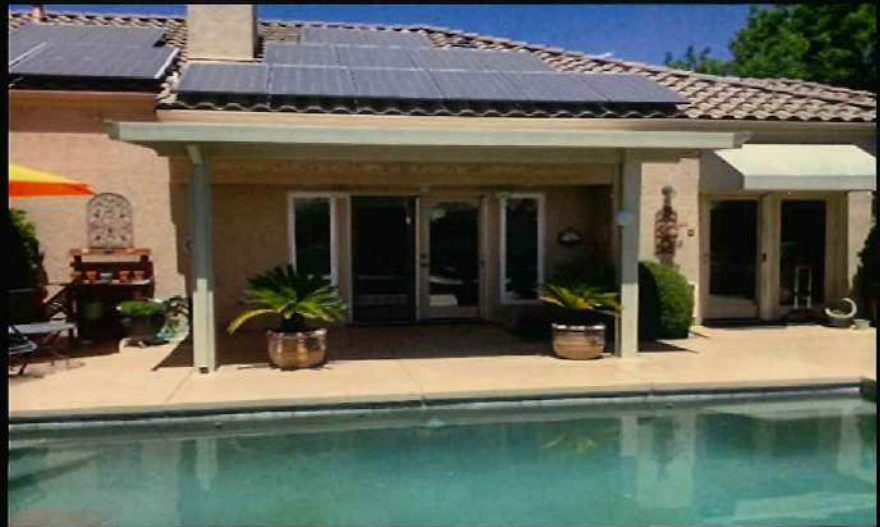
Classic flat pan cover wall attached with standard post wraps.
