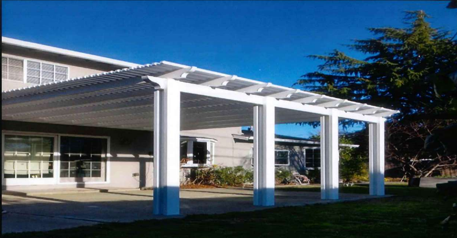
Classic Flat Pan Cover Eve attached. Standard post with a 3x8 for the post wraps.
