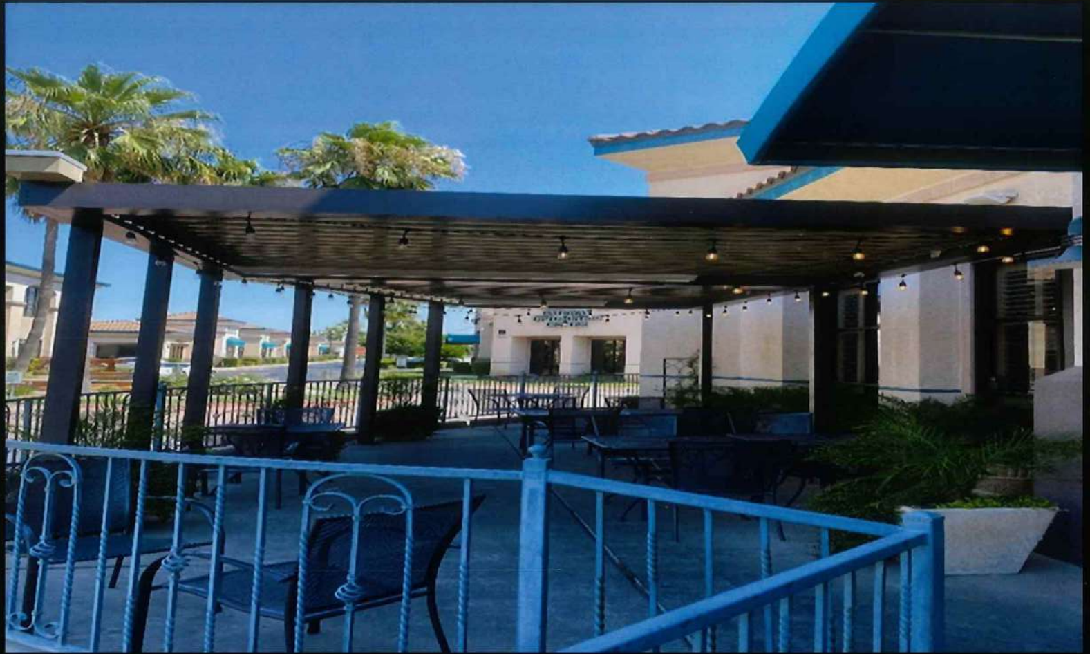
Equinox angled on one end with 7x7 post and 2x8 extrude frame 2 bays.
