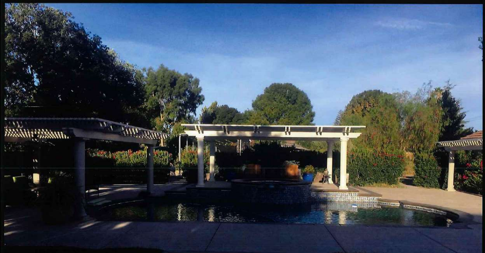
Ultra Lattice cover with 2x3 lattice tubes, double 2x6 rafters, double 3x8 beams and 10" round columns.
