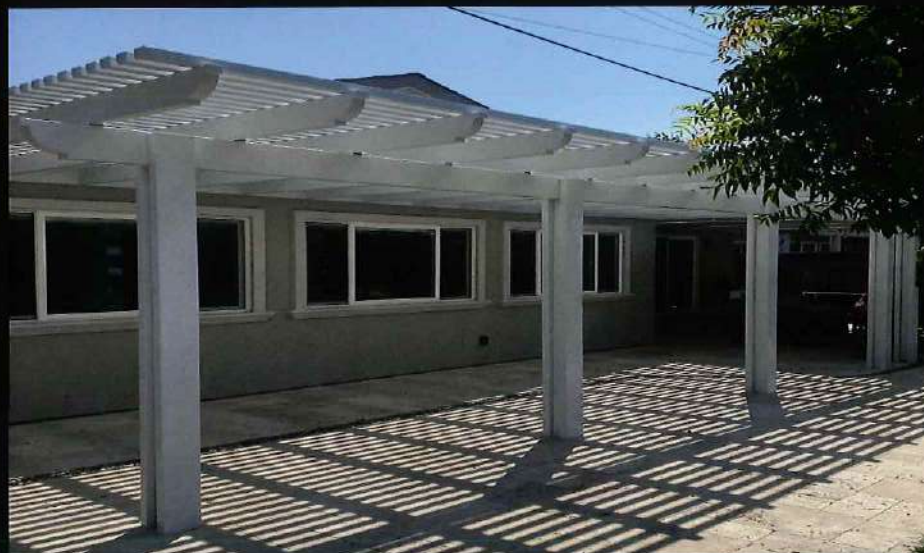
Ultra lattice cover with single 2x6 rafters, 2x3 tubes, single 3x8 beams with standard post wraps.
